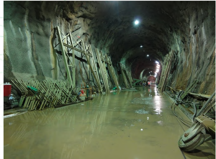
El Quimbo Hydroelectric Project - Underground diversion tunnel. Taken from
